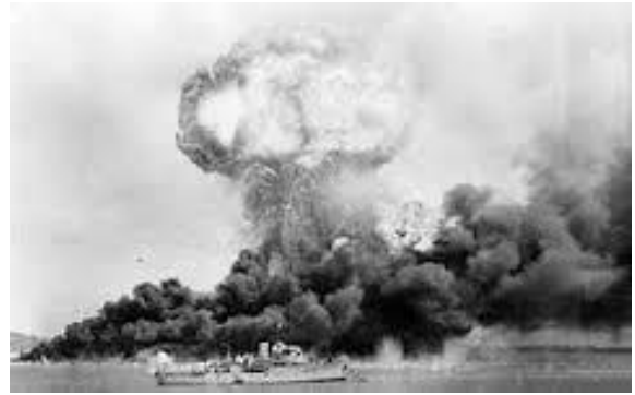
Fuel storage tanks burning in Darwin after the first Japanese air raid.
