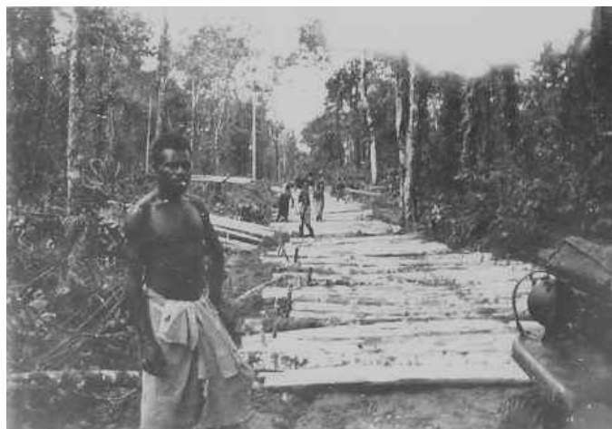
Roads covered with corduroy were spoiled by mud slurries.
