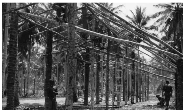
Workshop bays constructed from local coconut trees
