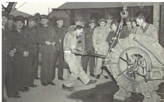
BRIG Field and party inspect vertical type of full circle mould after a tyre has been re-treaded at 8 th Advanced Workshop, AEME. (Photo AWMI)
