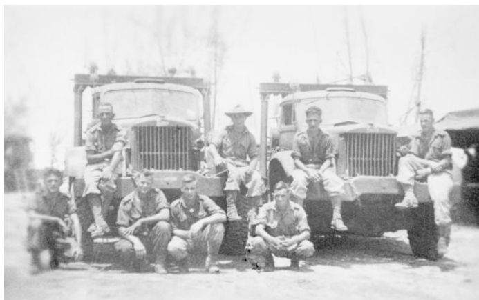
Recovery Group, 1 st Australian Beach Workshop, with Diamond T wrecker trucks after the invasion of Labuan off the Borneo north-east coast
